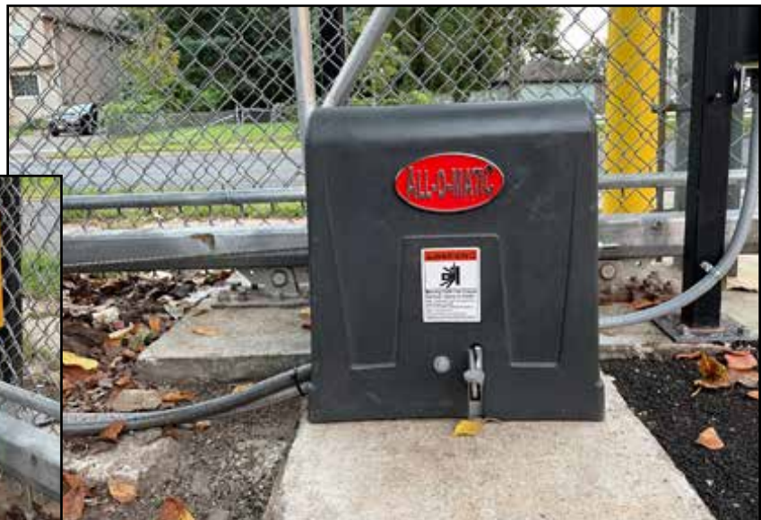
Shown SL90DC-C. Chain drive operator for sliding gates.
